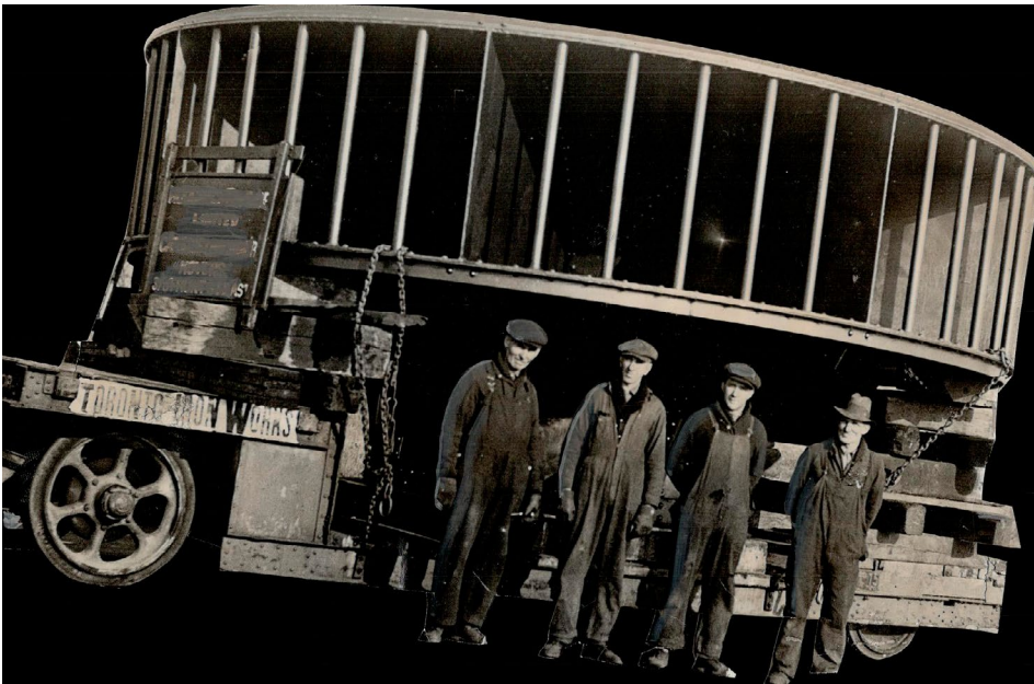
Original 1932 Toronto Star caption - "Torontonians will drink from this - the last piece of pipe in the city's new water supply system at Victoria Park Avenue [now R.C. Harris WTP]. It's enroute to its last resting place somewhere out in Lake Ontario."
