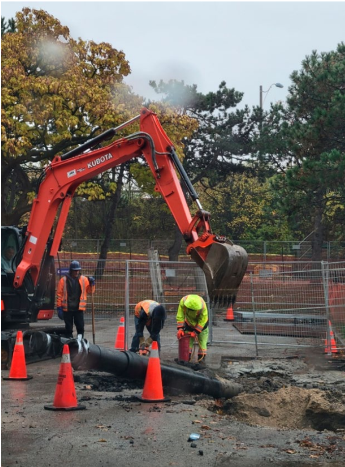
Receiving of the directionally drilled twin forcemain pipes.
