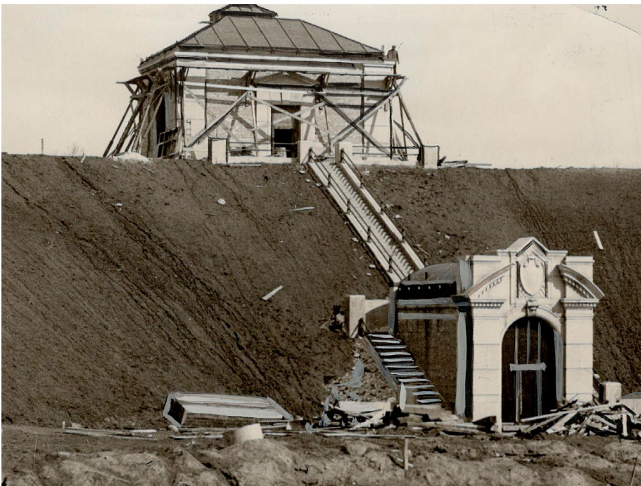
Toronto Star Photograph Archive: March 1931 "The new 50-million-gallon reservoir at St. Clair Avenue West and Spadina Road [now Winston Churchill Park] underwent a contractors' test last night and is now nearly ready for the city's use."
