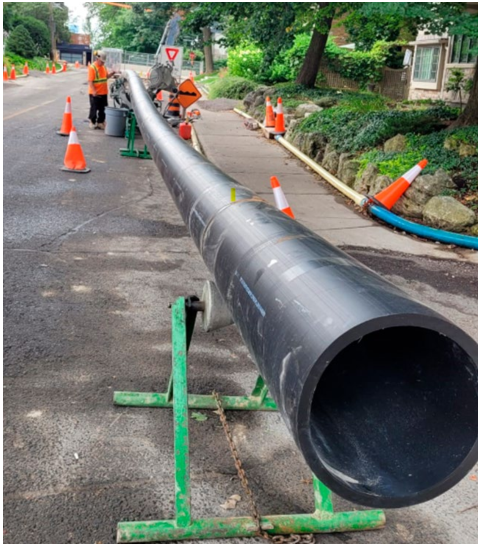
HDPE pipe to prior to installation.
